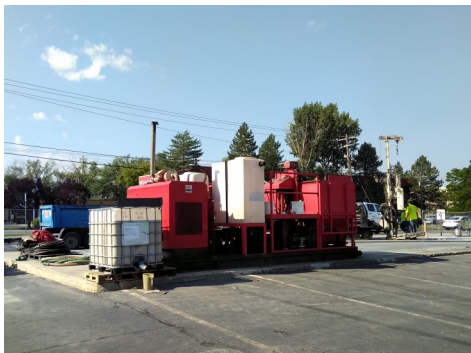
Pumping and Mixing Unit at the Site
